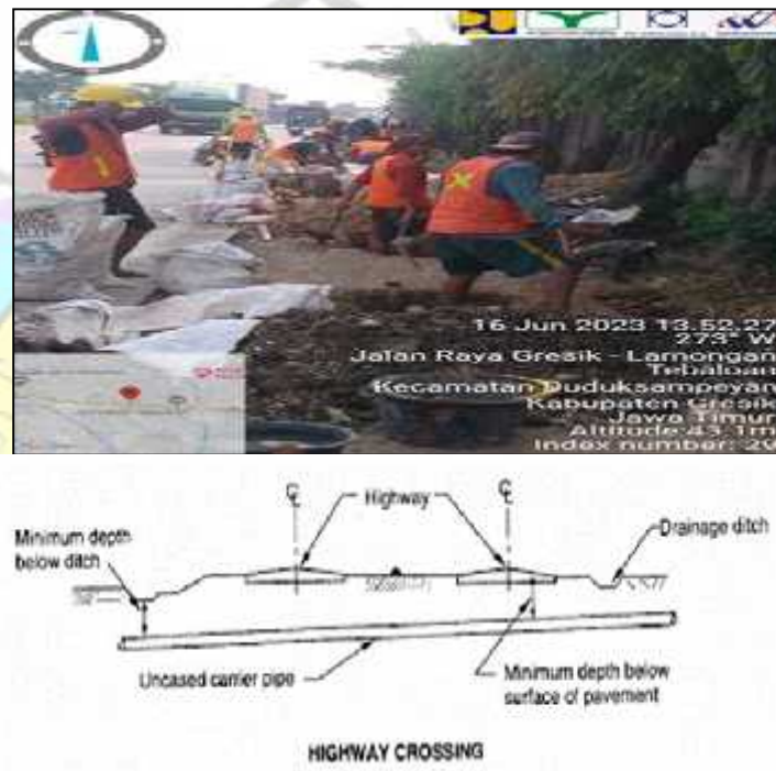
Gambar 2. 4 Metode Pekerjaan Borman (Boring Manual)
